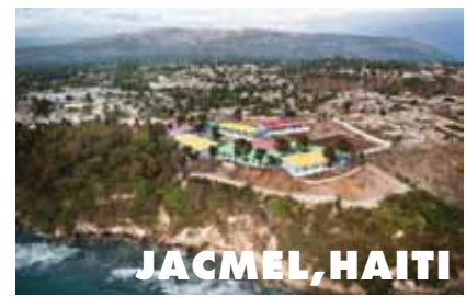
JACMEL, HAITI Operation USA teamed with Honeywell again to build a 40,000-square-foot school complex in Jacmel, a seaside town in Haiti savaged by an earthquake.
