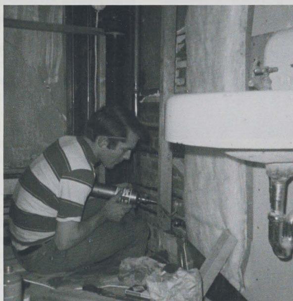
Colin S. Diver working on South End house, Boston, MA.
